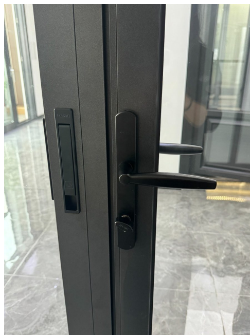
FINISHED LOOK Flush-pull and lever handles, installed
